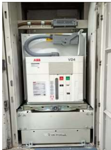
Retrofitting with cradle
